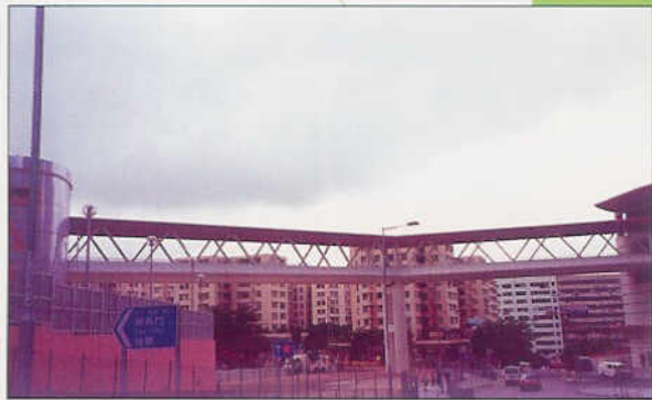
Yau Tong Redevelopment Footbridge Link Between Phase 1 to 5 油塘邨重建5期（連接第一期至第五期）行人天橋上蓋
