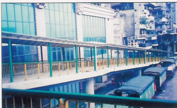
Footbridge Cover Adjacent to Western Recreation Centre, Sheung Wan 西區室內運動場側行人天橋上蓋
