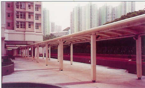
Podium at Yau Tong Redev. Phase 5 油塘邨重建5期平台
