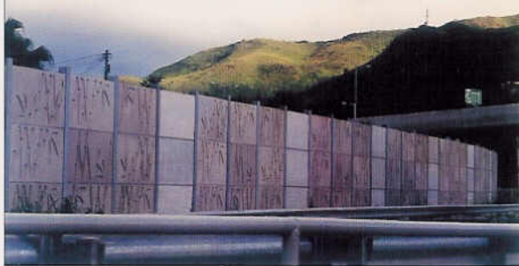
Concrete Feature manufactured using GRP Waffle Mould 三號幹線石屎裝飾
