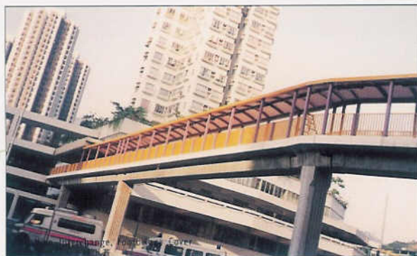
Tsuen Wan Interchange, Footbridge Cover 荃灣交匯處行人天橋上蓋
