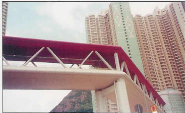
Yau Tong Redevelopment Footbridge Link Between Phase 1 to 5 油塘邨重建5期（連接第一期至第五期）行人天橋上蓋
