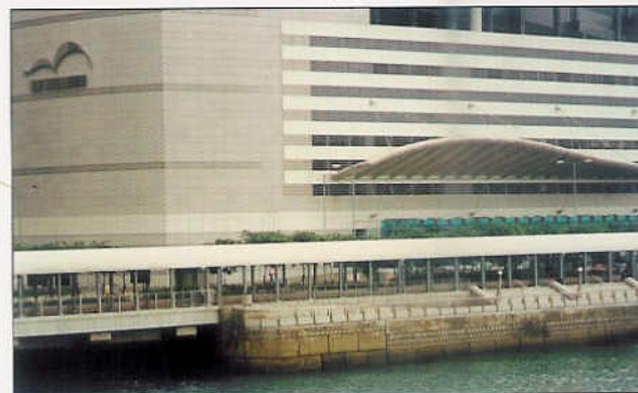
Walkway Cover adjacent to Hong Kong Convention and Exhibition Centre Extension Phase 香港會議展覽中心行人路上蓋
