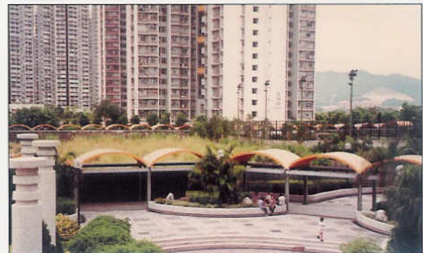
Tin Shui Wai Walkway Cover 天水圍行人路上蓋
