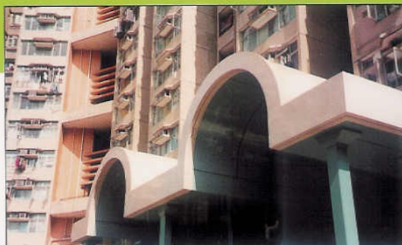
Tai Wo Estate Walkway Cover 太和邨行人路上蓋
