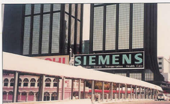
Walkway Cover adjacent to Hong Kong Convention and Exhibition Centre Extension Phase 香港會議展覽中心側之行人路上蓋
