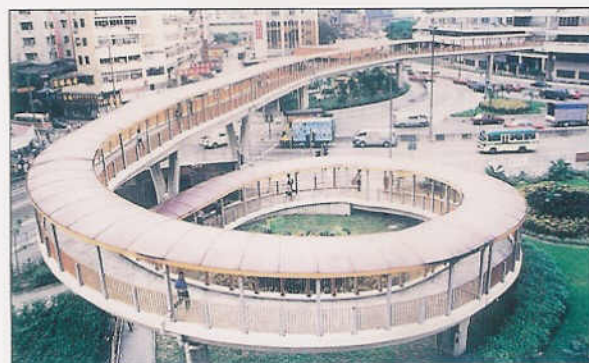
Tsuen Wan Ferry Pier, Footbridge Cover 荃灣碼頭行人天橋上蓋
