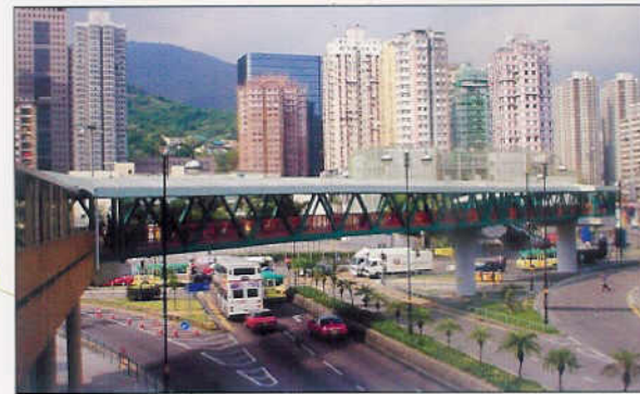
Tsuen Wan Footbridge Cover (To CityHall) 荃灣大會堂行人天橋上蓋
